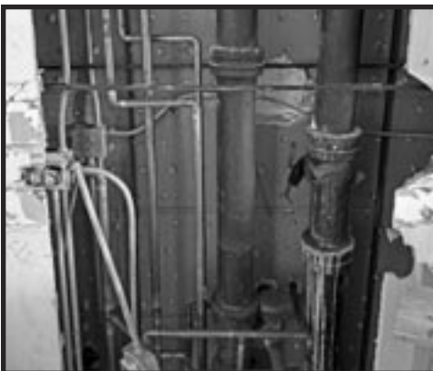
➤ Pictured here are typical existing conditions in a plumbing wall.
