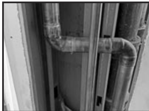
➤ Shown here is new copper piping being installed.
