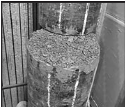
➤ Shown here is the inside of a hot water pipe that has been sandblasted.
