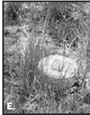
E. Waste Cleanout
