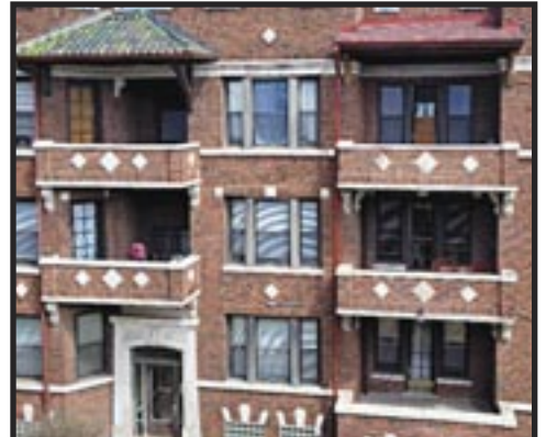
Cantilevered balconies
