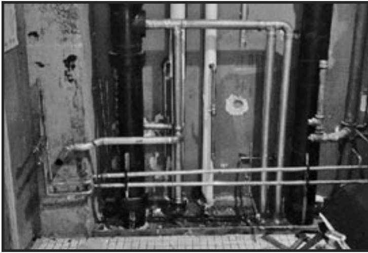
Plumbing Piping Replacement In Apartment Building
