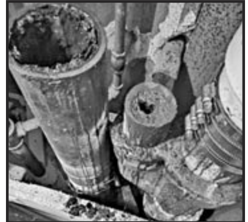
Shown here is an image of grease buildup in kitchen waste piping that undergoes regular maintenance.
