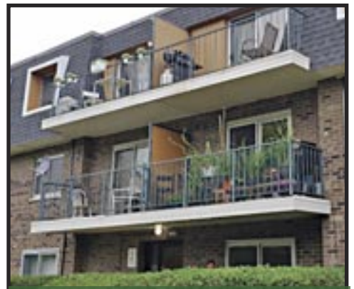
Cantilevered balconies with metal handrails
