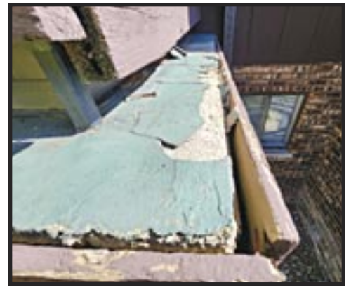
Shown above is rotted wood at a balcony location.
