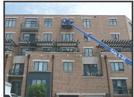
➤ Shown here is the installation crew using their articulating boom lift to place a new window.
