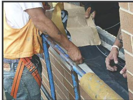
➤ Window perimeter sealant was installed around the interior and exterior of the windows to limit air leakage through the gap between the window frame and building.
