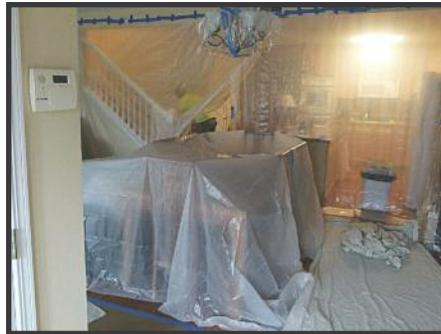
➤ Shown here is the inside of a condo unit protected with plastic covering to avoid any damage during window replacement work.
