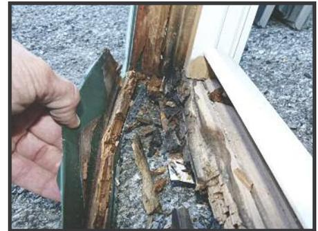
➤ Shown here is one of the window sills that had rotted wood from water penetration and caused a potential hazard of a window falling out.
