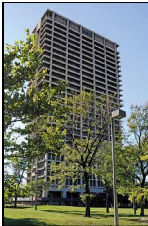
➤ Shown here is University Hall at UIC - in foreground is the location of the geothermal well-field.
